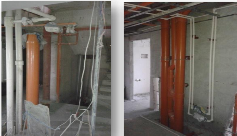
d Storm Drain Line And Water Line
