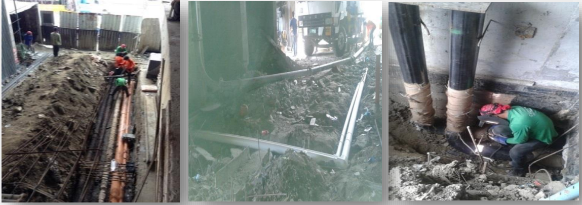
a Pipe laying for Storm drain, Water line and Sanitary line, Air-con drain, Fire Protection pipe at Ground Floor.
