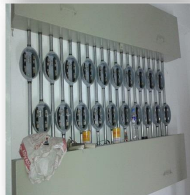
4F to 15F Meter Center & Wiring Installation at Electrical Room
